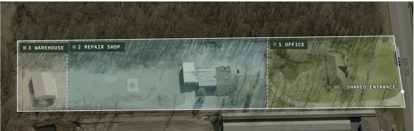
AERIAL OF THE SITE. ZONE BOUNDARIES ARE INDICATIVE, NOT SURVEYED.
